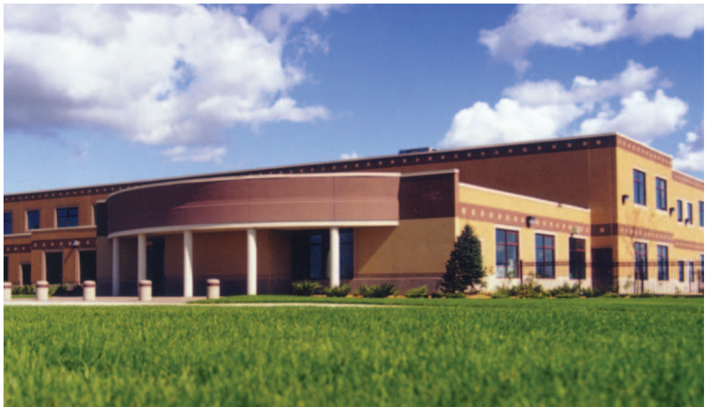
A recent school construction project was completed using Scott Systems Thin Brick with tilt-wall construction.
